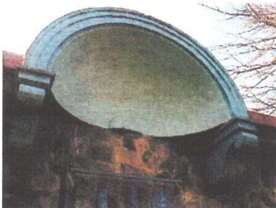
Portico of residence. © DPIPWE July 09.
