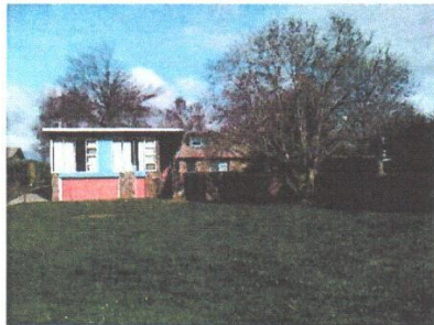
Rear apartment and storage area under podium lawn. ©DPIPWE July 09.
